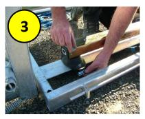
Using bolts with square washers, clamp the load bars to the Weigh Frame with the ridge of the square washer facing outwards. Put on the flat washer, spring washer, and nut loosely until checked for squareness. Tighten bolts using 18mm and 19mm ring spanner. These load bars can now stay permanently on the Weigh Frame.
